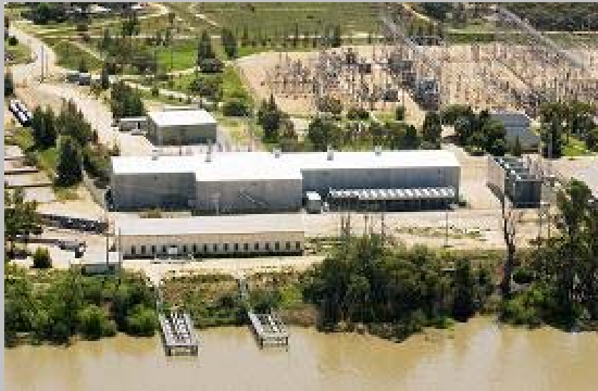
Red Cliffs Converter Station
