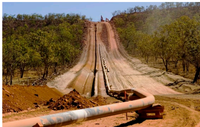
STRINGING THE BONAPARTE PIPELINE 2006
