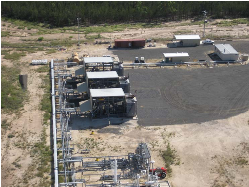
Plate 1: Kogan North Central Gas Processing Facility
