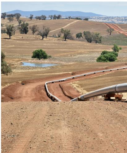
Example of a pipeline under construction, prior to being lowered into the ground.
