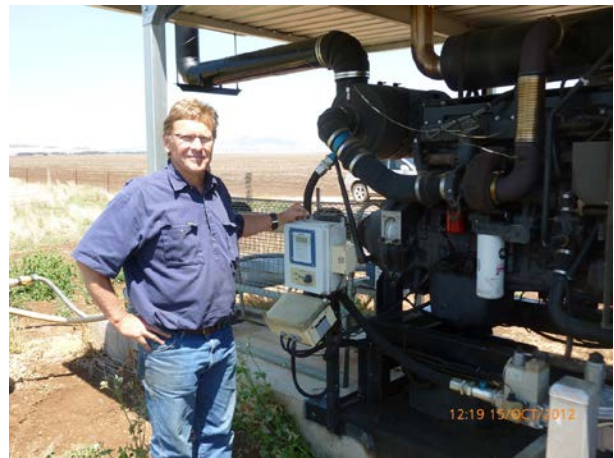
Figure 1: David Ronald in front of his bore pump powered by compressed natural gas.
