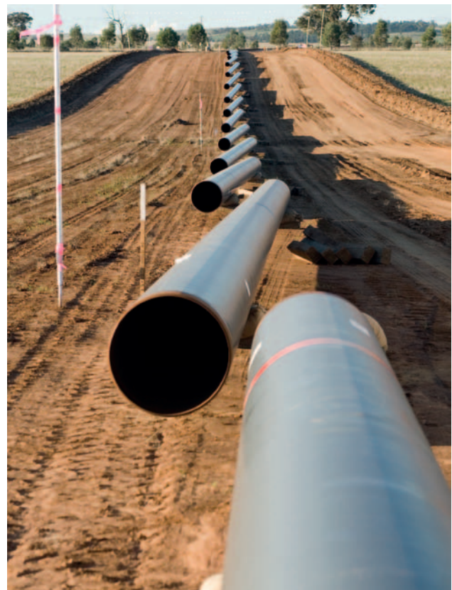
Capacity expansion on the Moomba to Sydney pipeline, Young looping, NSW.
