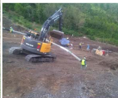
Repairing the pipeline
