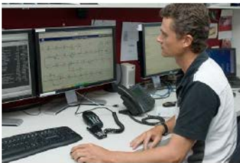
Darwin pipeline control centre
