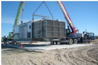
Installing the compressor station at Marsden
