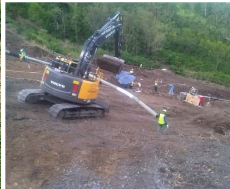
Repairing the pipeline
