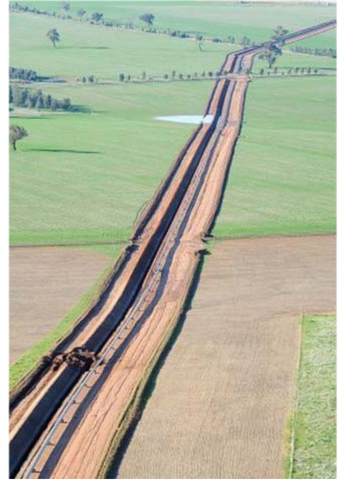
Pipeline prepared for lowering
